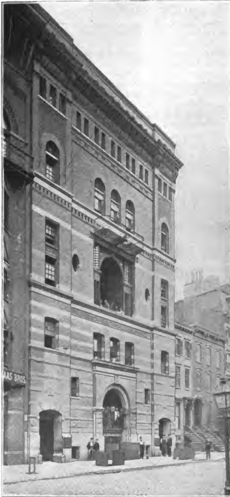
EDISON ELECTRIC ILLUMINATING CO., 26TH STREET, BETWEEN BROADWAY AND SIXTH AVENUE.
